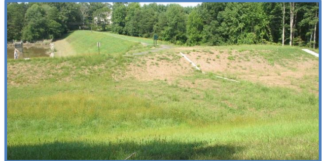
Completed project shortly after construction with the two cutoff walls installed.
