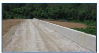
A parapet wall was constructed across the top of the dam embankment during the rehabilitation project to raise the top of the dam to the designed elevation.
