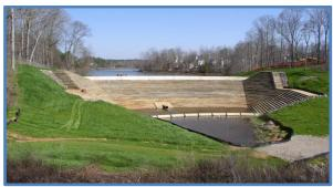
Rehabilitation of the dam included installing a roller compacted concrete spillway over the top and down the back slope of the dam.
