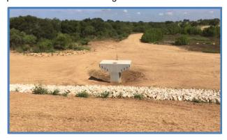
A new concrete inlet tower and a 42-inch diameter reinforced concrete conduit were installed during rehabilitation of the dam.
