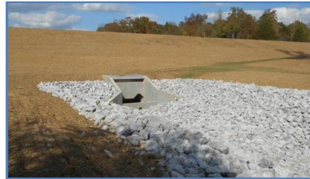
A new outlet channel and impact basin was constructed as part of the rehabilitation project.
