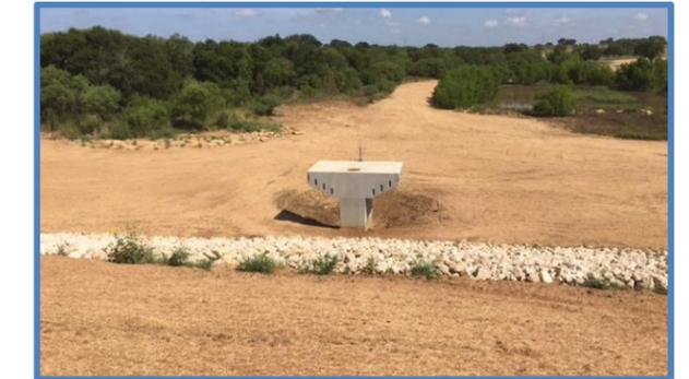
A new concrete inlet tower and a 42-inch diameter reinforced concrete conduit were installed during rehabilitation of the dam.
