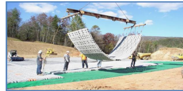
Sections of the auxiliary spillway were covered with articulated concrete blocks to prevent surface erosion.
