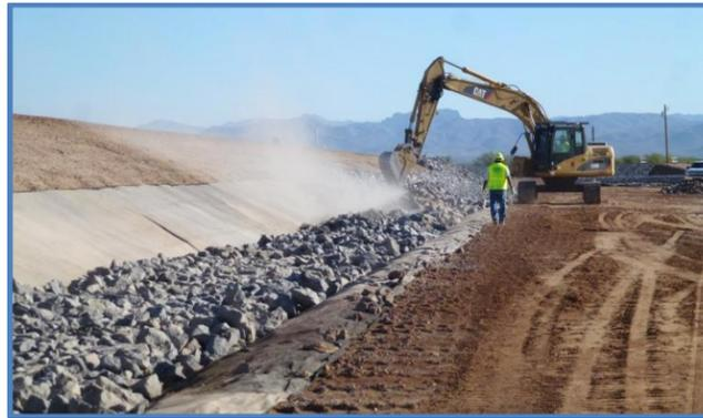
Rip rap rock was placed for erosion protection for the auxiliary as part of the rehabilitation project.
