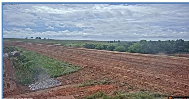
The height of the dam embankment was raised 6.3 feet during rehabilitation. A new inlet tower and principal spillway conduit was also installed.
