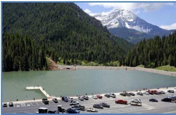
Tibble Fork Dam after completion of rehabilitation project.
