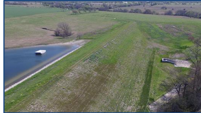
East Fork Above Lavon Dam No. 2A after rehabilitation project was completed.
