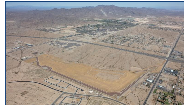
Aerial view of White Tanks No. 4 Flood Retarding Structure
