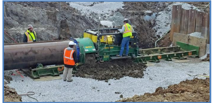
Installation of a new principal spillway pipe on Dam No. 16
