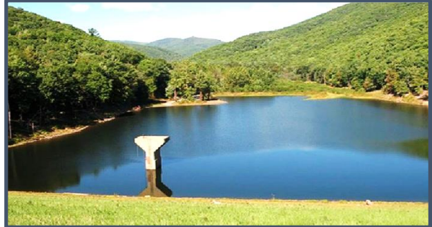
The current dam does not meet current dam safety standards.
