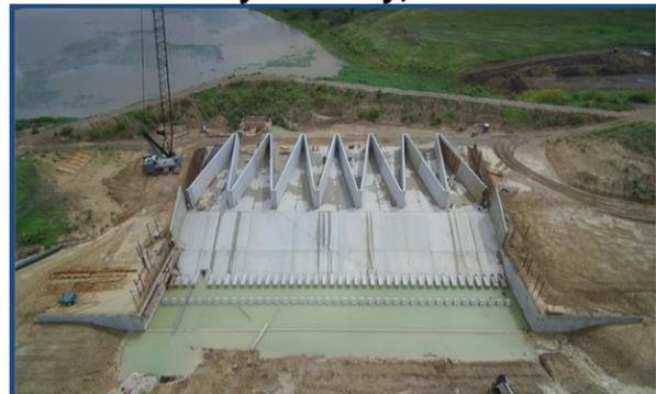
A labyrinth weir was installed to replace the current earthen spillway during rehabilitation.
