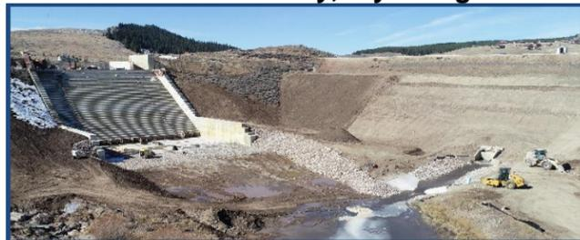
A concrete labyrinth spillway and mass concrete spillway chute and stilling basin were installed as part of the rehabilitation project.
