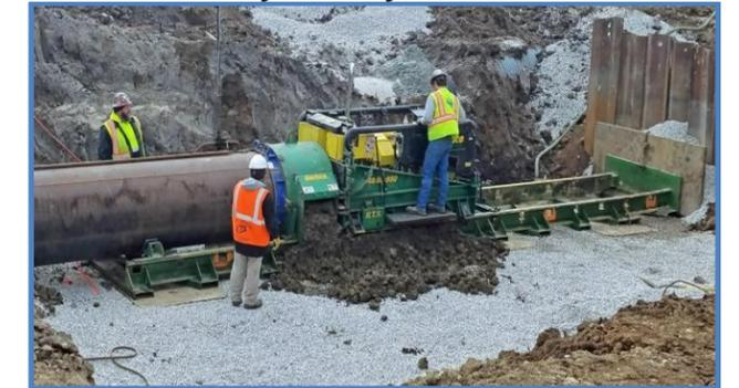
The spillway pipe was replaced during the rehabilitation of Dam No. 16.
