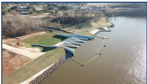
A concrete labyrinth weir auxiliary spillway was constructed over the embankment during the rehabilitation project.
