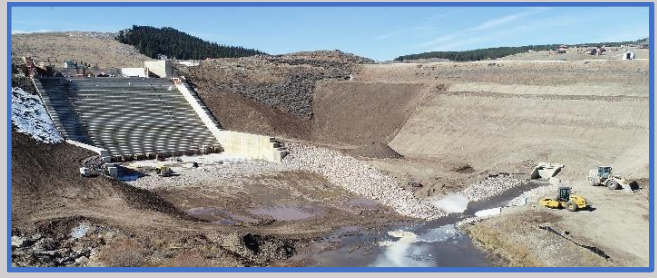
Dull Knife Watershed Dam, Johnson County, Wyoming
