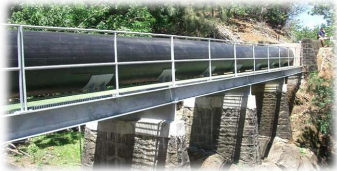
The Lower Hamakua Ditch Watershed Project on the island of Hawaii help rebuild and repair a water distribution system that had been built by sugar companies from 1900 to 1910. The 15 miles of open ditch and 10 miles of tunnel provide irrigation water distribution to 8,000 acres of agricultural lands. This flume replaced an existing one that had deteriorated.
