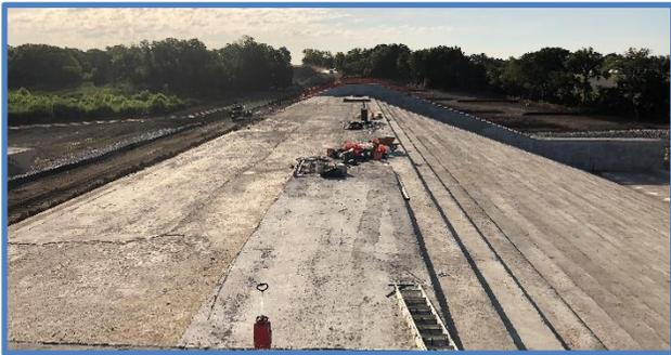
A roller compacted concrete spillway was constructed over the top of the dam during rehabilitation to replace the current earthen spillway.
