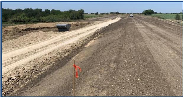
The height of the dam is being raised and rip rap rock is being added to the front slope for wave protection.
