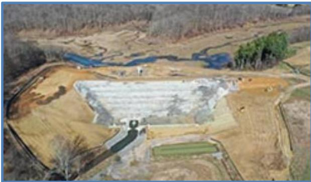
A roller compacted concrete spillway was constructed over the top of the dam during rehabilitation.
