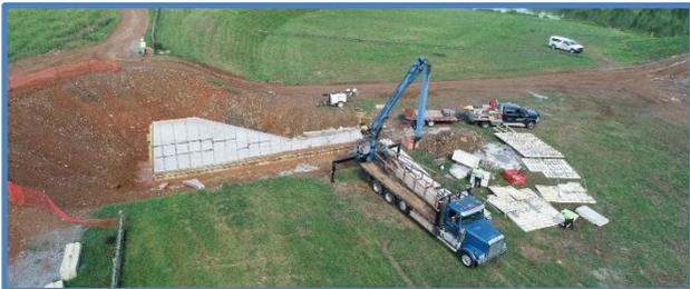
A concrete cut off wall was constructed in the spillway.
