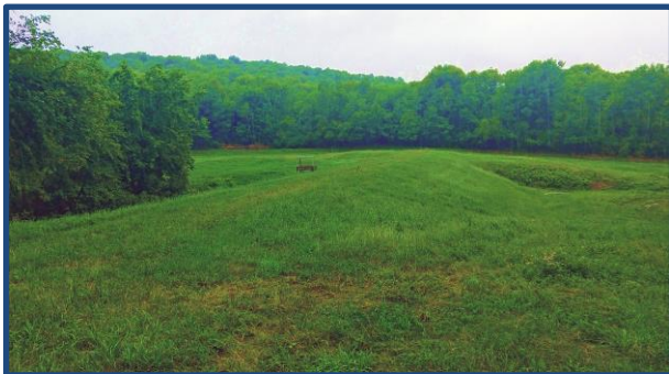
Dam in 2021 before rehabilitation
