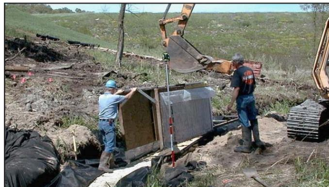
Tile drain being replaced in the West Fork Dam No. 1 (Jersey Valley Dam) in Vernon County as part of operation and maintenance work.
