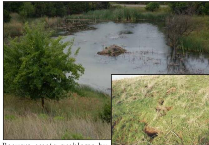
Beavers create problems by damming up areas below the dam and backing water over the outlet pipe restricting flow. They also burrow into the dam which can cause serious erosion problems and they often plug up the inlet tower.
