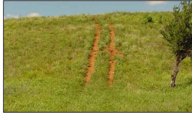
Cattle trails on dams can lead to serious erosion problems if not corrected.
