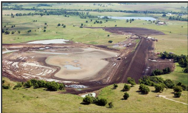
Double Creek Watershed Dam No. 3 during rehabilitation construction.
