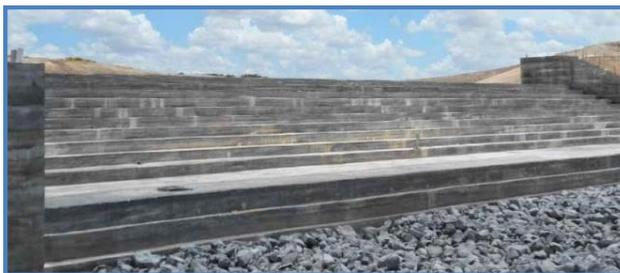
The original earthen auxiliary spillway for the dam was replaced by a wider roller compacted concrete (RCC) spillway during the rehabilitation project.
