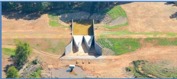
Rehabilitation of the dam included constructing a 54-foot wide concrete chute auxiliary spillway with a two cycle labyrinth weir over the top of the existing dam
