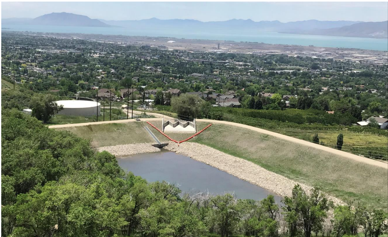
Battle Creek Dam - looking downstream at the auxiliary spillway (labyrinth weir) to Pleasant Grove City
