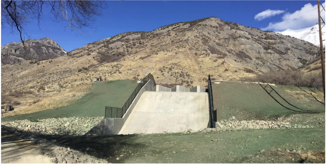
Battle Creek - looking upstream - auxiliary spillway
