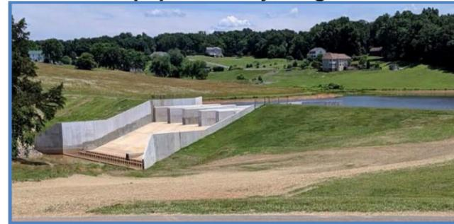
A six-cycle structural concrete labyrinth spillway was constructed over the embankment.
