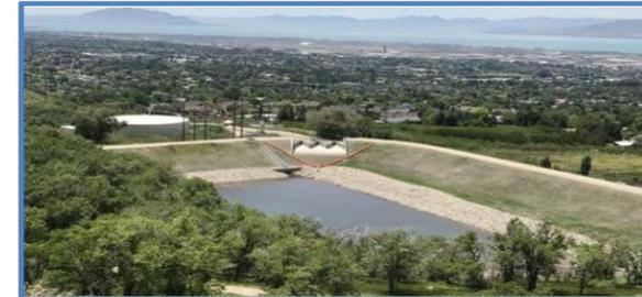
Rehabilitation included raising the crest of the dam by two feet and replacing the auxiliary spillway with a concrete labyrinth weir.
