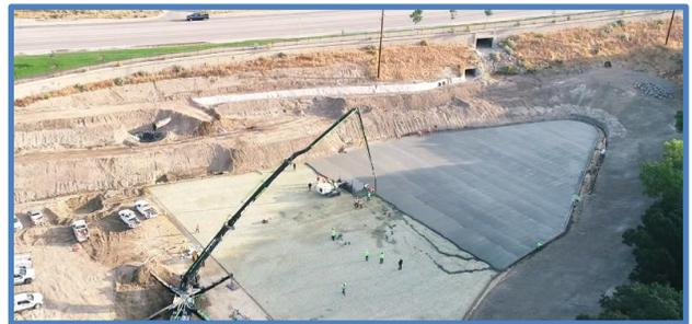
The upper end of the debris basin is being covered with concrete for easier sediment removal.
