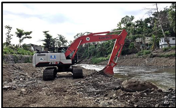
Stream restoration work in Puerto Rico after hurricane damage
